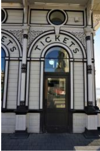
Ticket Office Street Level Access - IN Door Closed
